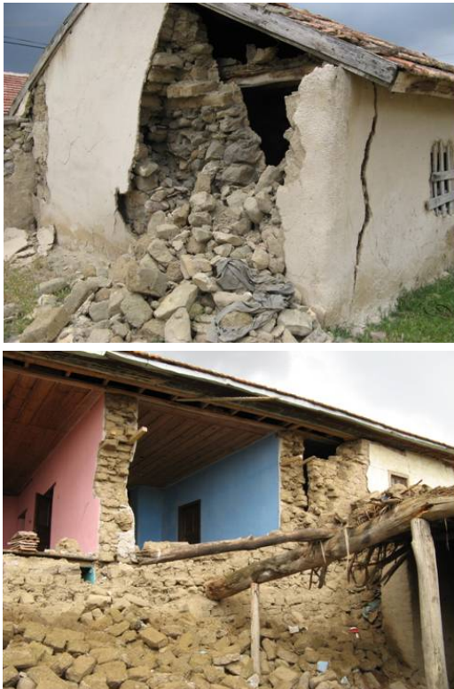
Fig. 9. Examples of heavily damaged masonry buildings.
