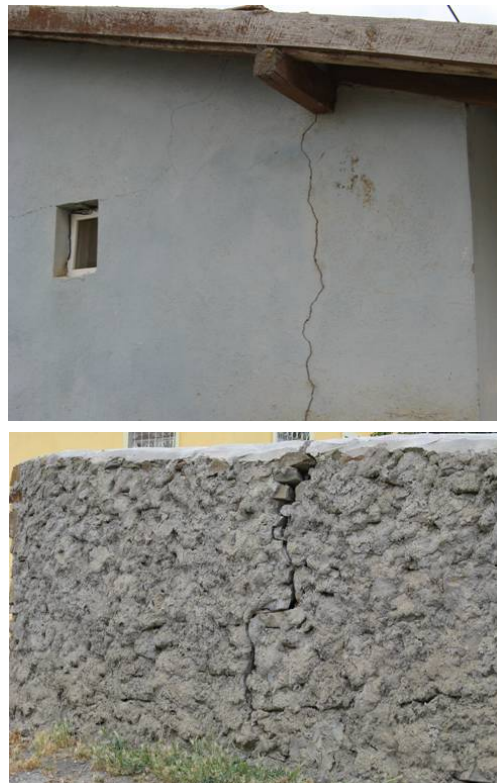
Fig. 15. Examples of shear cracking under vertical shear force on the structural walls.
