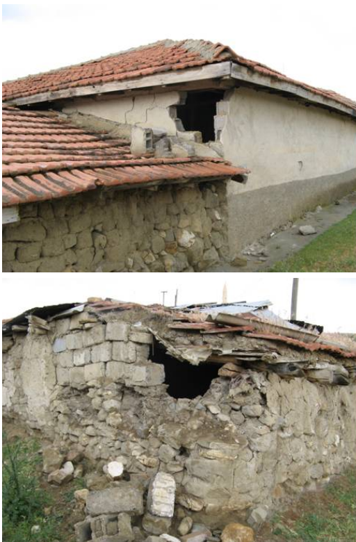
Fig. 10. Examples of failure of masonry building corners.
