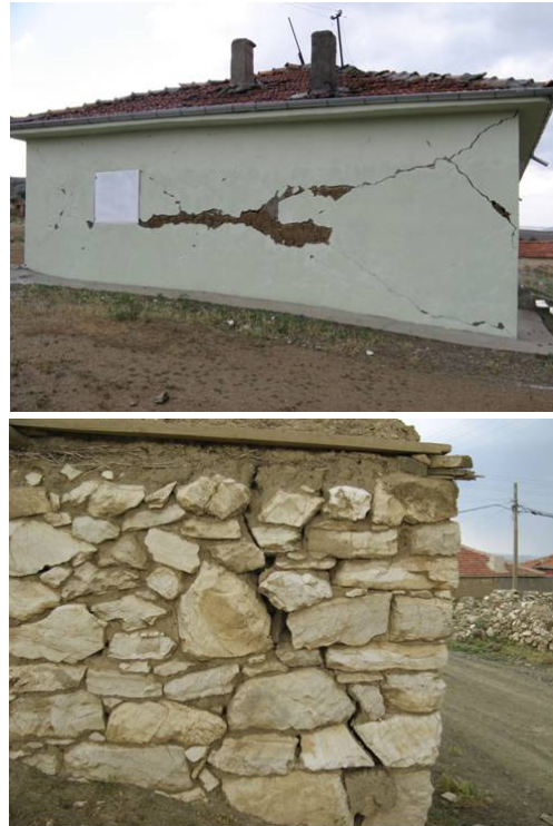
Fig. 14. Examples of diagonal shear cracking on the structural walls.
