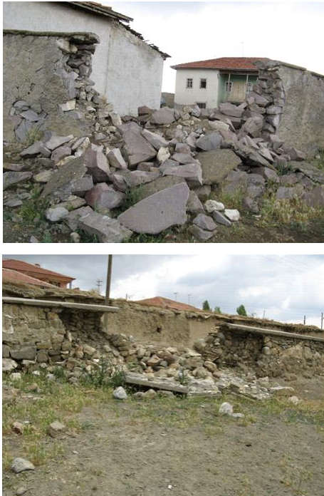
Fig. 19. Examples of damages on the stone masonry fences.
