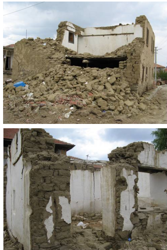
Fig. 8. Examples of completely collapsed masonry buildings.
