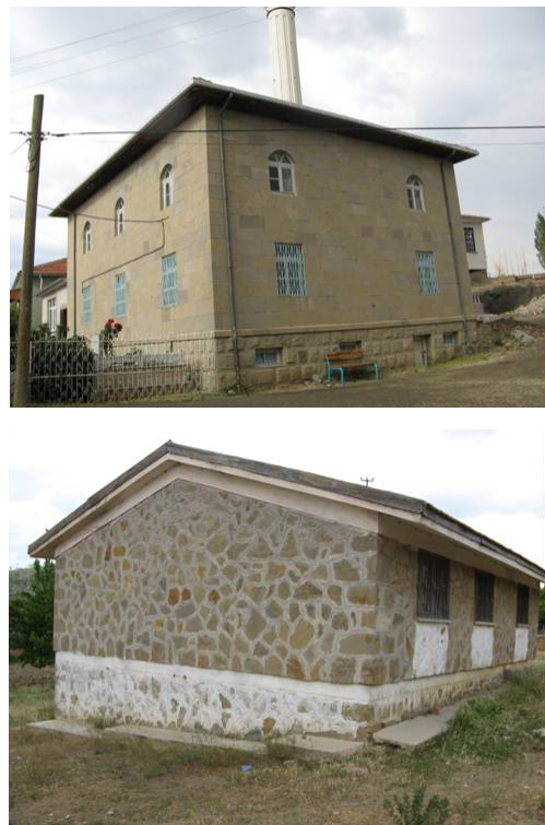
Fig. 22. Examples of undamaged masonry structures.
