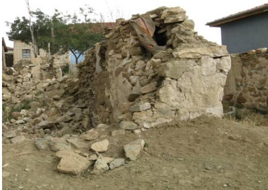
Fig. 13. A masonry wall with cavity and mud mortar.
