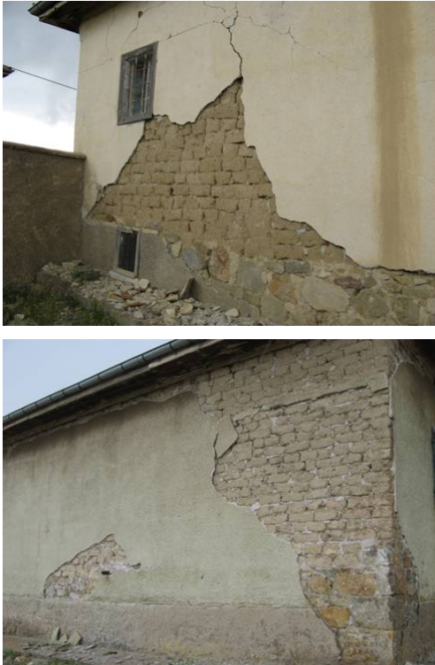
Fig. 16. Examples of out-of-plane failure (swelling) on the structural walls.
