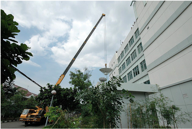
Fig. 19. The term “VSAT” (Very Small Aperture Terminal) may be misleading: considerable logistical effort was involved in the deployment of both the sensor and center to center communication links.
