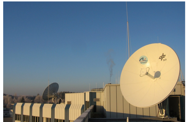
Fig. 13. The two VSAT antennas on the roof of BMKG headquarters in Jakarta (top) and on a building of DLR in Oberpfaffenhofen (bottom).
